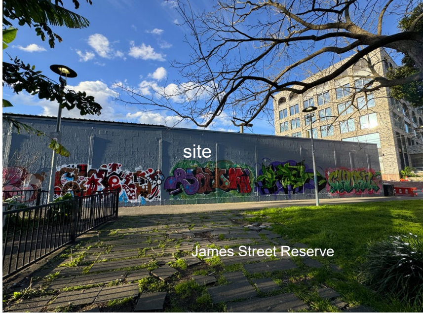
existing southern boundary wall of the site
