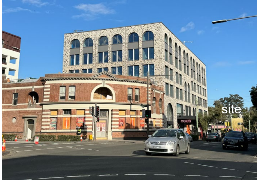
Surry Hills Village development to east of site
